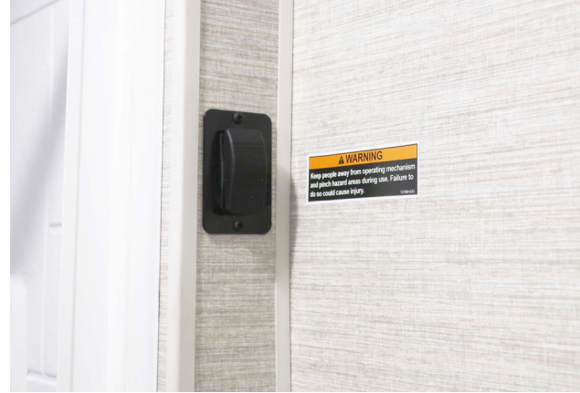
Murphy Bed Switch (Located near shower)
